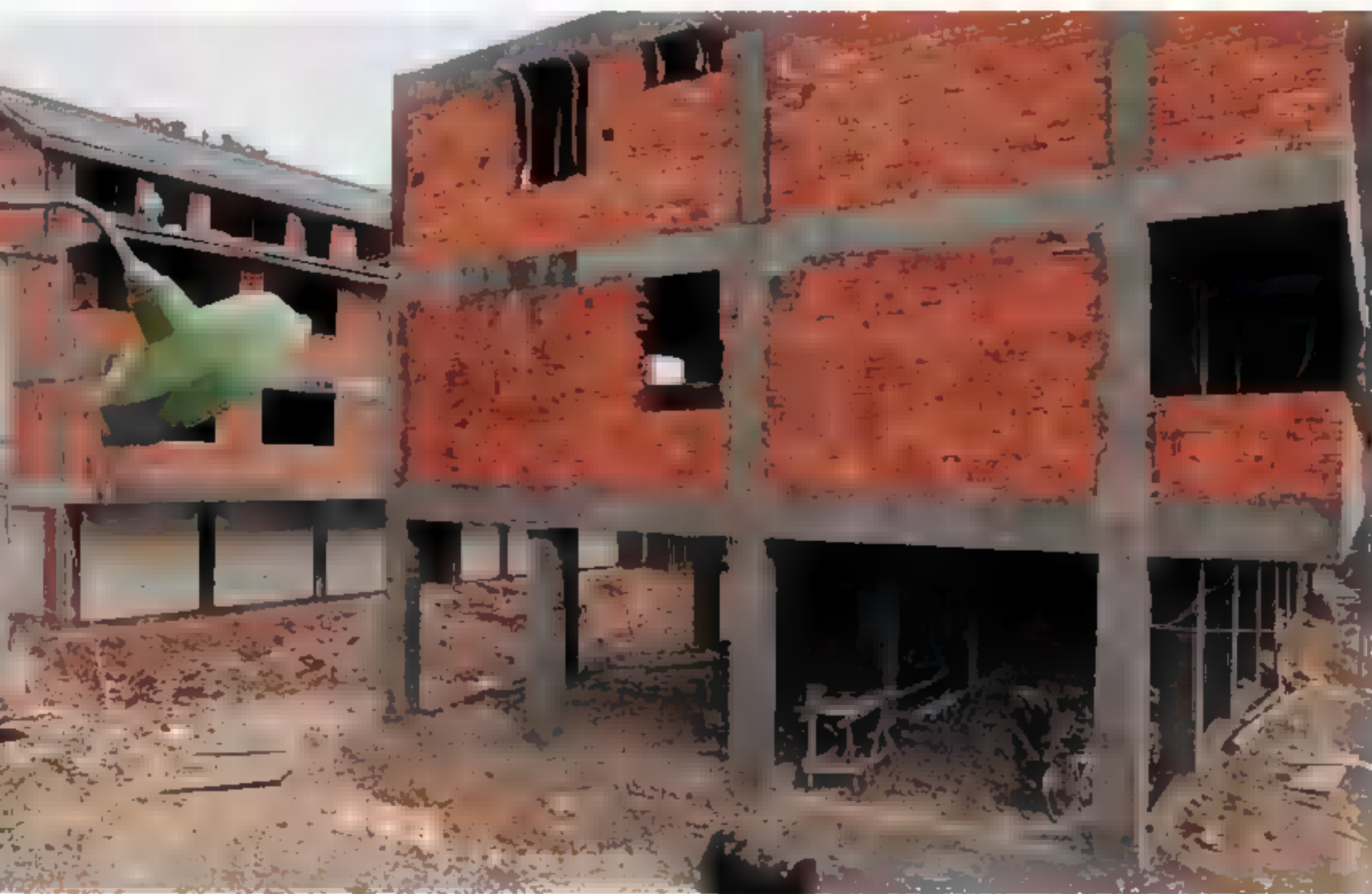
FEBRUARY 2006: SHELL FINISHED
